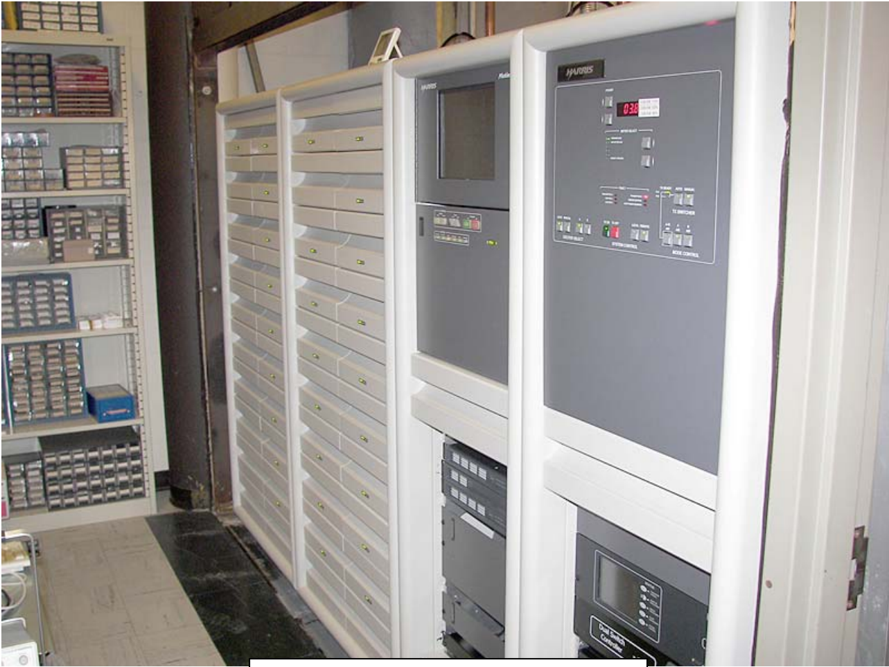
On air Transmitter
