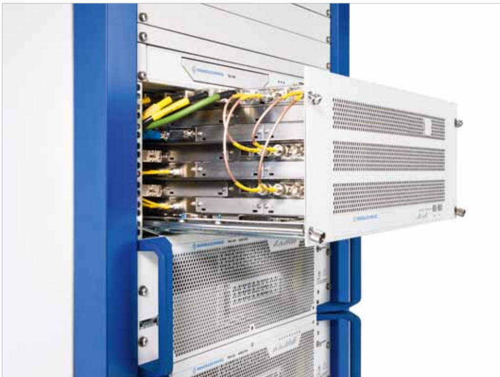
R&S®TMU9 with 1.14 kW DTV output power in dual drive.
